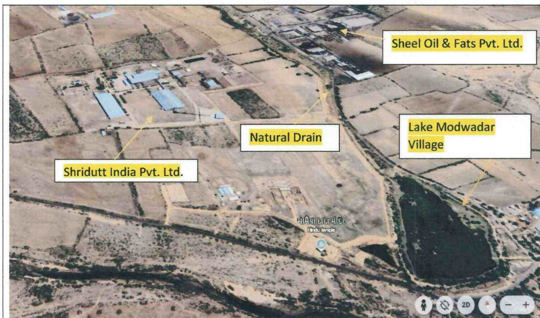
Figure:1 Google earth image of the unit and adjoining area.
